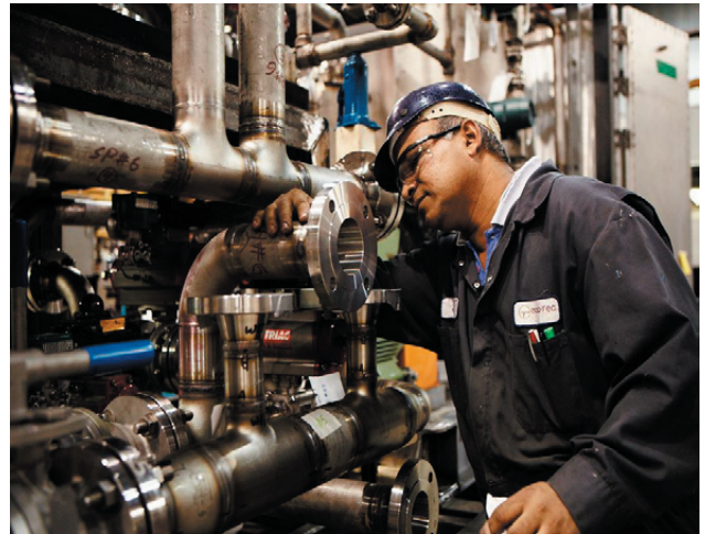
Eco-Tec staff putting final touches on equipment.
