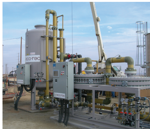
A 7,000 BPD Spectrum Plus Micro Media Filter feeding a SAC/WAC brine ion exchange softener supplying a steam generator.
