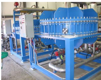
An Eco-Tec RecoPur Water Softener similar to the one to be installed at the Holmes Western Oil Company in Taft, California.
