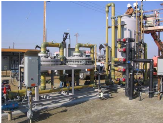
Figure 2: Short Bed Softening System 200gpm (6,857 bpd)
