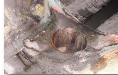
Lean/Rich Heat Exchanger
